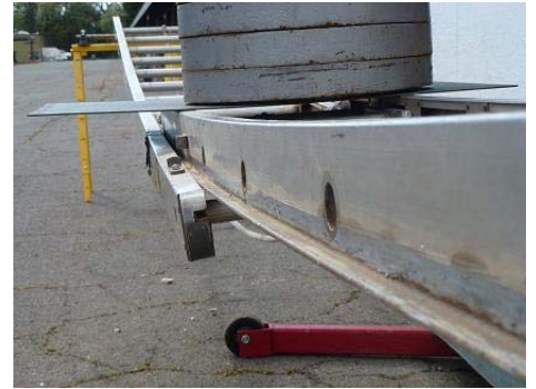
Why do we do ladder testing? To find ladders like this one above and to remove them from service, before someone gets hurt from it failing on the fire-ground.
